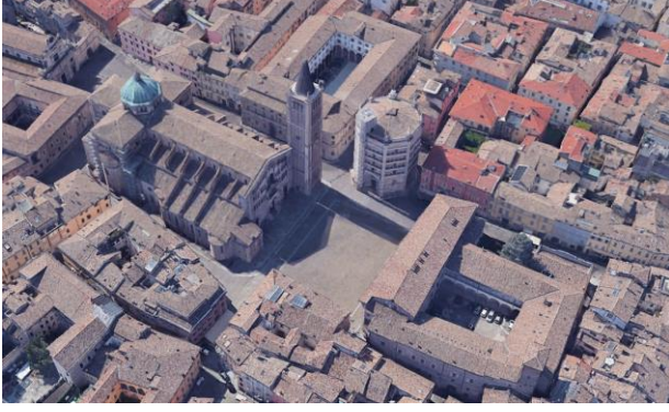
Fig. 1. Aerial view of Piazza Duomo in Parma, Italy (from Google Earth).
